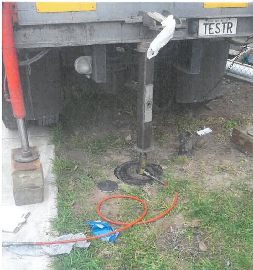
Figure 1 - Test set up. Photo shows load of 26.9kN applied hence the deformation in the service box.
